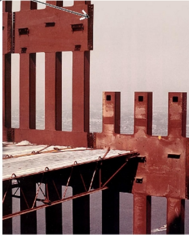
Construction of the World Trade Center Perimeter Column Panels Three Full Columns Connected by Three Spandrels
