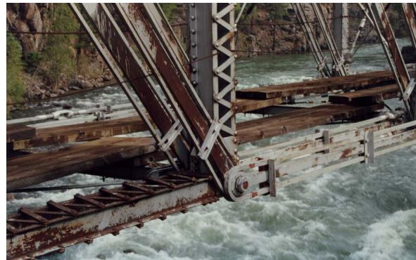
A Pinned Connection
