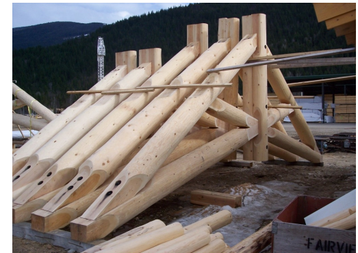
Mortise and Tenon Joint on Trusses For Log Homes
